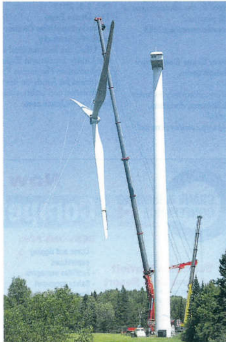
Grues Guay of Montreal employs a Liebherr LTM 11200 (left and above) on a wind project at Saint-Ferréol-les-Neiges, Que.
