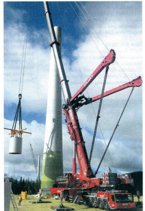
Grues Guay of Montreal employs a Liebherr LTM 11200 (left and above) on a wind project at Saint-Ferréol-les-Neiges, Que.
