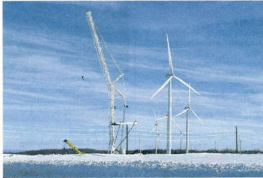
Liebherr LTM 11200-9.1 works in winter on a wind farm in upstate New York. Photo courtesy of Northern Crane Services
