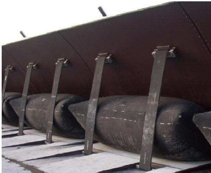
Figure 16: Example of an Inflatable Weir Structure
