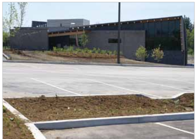
Bioretention gardens in the parking lot of the Oak Ridges Community Centre.
