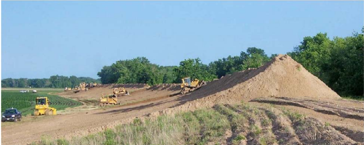
Figure 3. Illustrative picture of UMR sand levee with incomplete push-down after 2008 flood fight.
