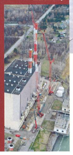
ate in 2013, Sorel-Tracy, Quebec province, Canada-based Guay Inc. was called on to develop an engineering and lifting plan and provide the cranes to dismantle four chimneys that stood about 465 feet tall. The cranes would need to lift 75,000 pounds at a 105foot radius and would need to be able to move quickly between each chimney with the boom fully erected.
